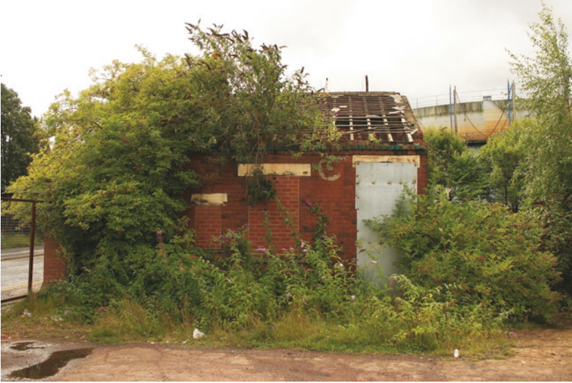
Fig. 2.3 Cottage in summer, 2009. Photograph by the author
