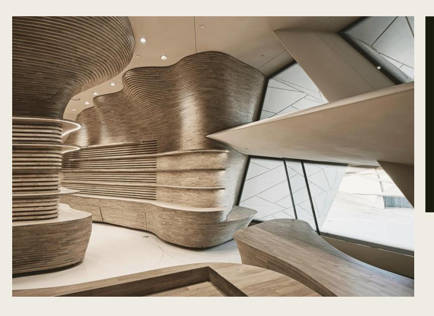
No less than **40,000** individual pieces of sustainably sourced European oak were designed with 3D modelling software. Each piece, CNC-cut (Computer Numerical Control) in Italy is entirely unique, fitting only with its exact complementary piece. The site assembly was an engineering and assembly challenges that was skilfully executed on-site by Italian master carpenter, Claudio Devoto and his team of artisans. The 40,000 pieces were inserted in numbered order into a rib-like steel structure.
