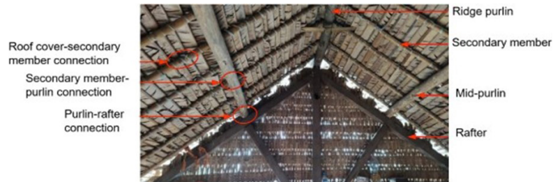
Figure 2. Members and connections in the roof structure
