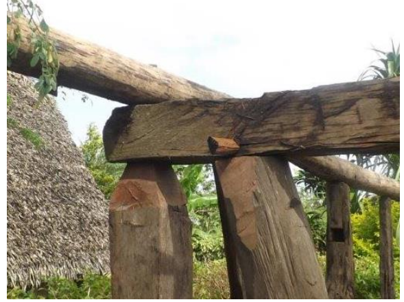
Figure 7: Example of traditional pegged mortise and tenon connection (image from Care International)
