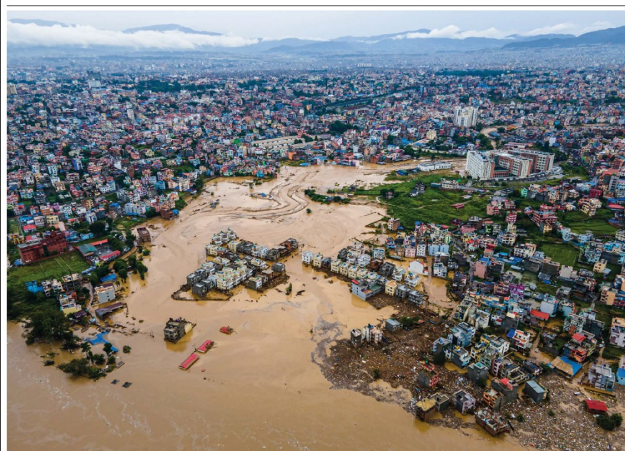
Figure 1 | Flooding of the Nakkhu River in Lalitpur, Nepal. Record rainfall in late September caused extreme flooding of the Nakkhu River, a small river in the Kathmandu Valley. The water flowed over the embankments that are designed to mitigate the risk of flooding, seen here in the middle of the river.
