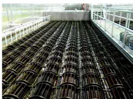
C. Algae Wastewater Treatment System - Algaewheel Technology (http://www.todayfacilitymanager.com/facilityblog/wp-content/uploads/algaepac-1-1024x768.jpg)
