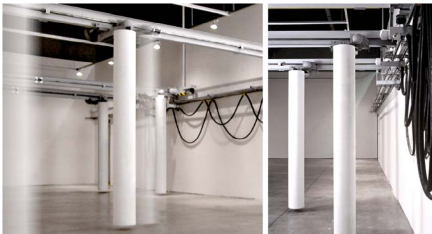
Fig 3: Shuffle (Los Angeles, California, USA) by Jones, Partners: Architecture, 2003. This installation at the Southern California Institute of Architecture demonstrates a prototype system for re-configurable architectural space-making elements. In this case, three columns can be repositioned in order to allow individuals to create different architectural relationships within the gallery space. (Image courtesy of Jones, Partners: Architecture).
