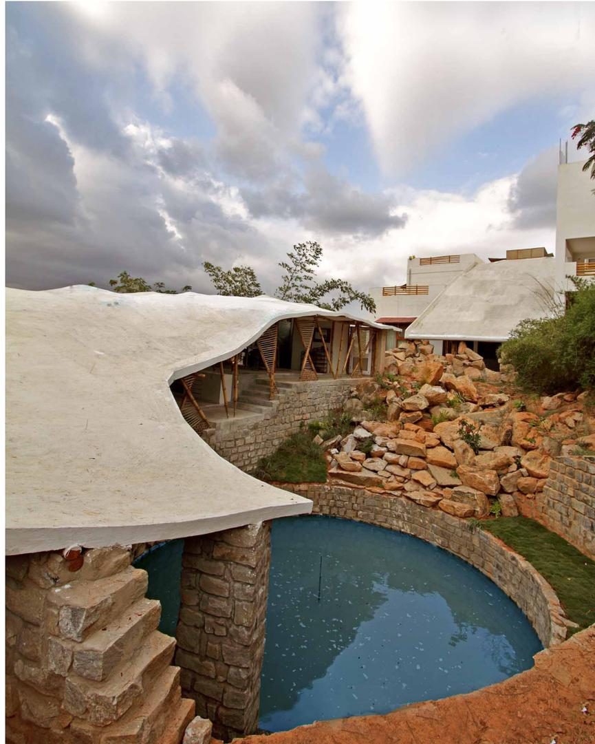
Figure 8: The criss-crossed bamboo columns hold the fabric roof.
