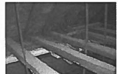
Plate 5 Moray House, Edinburgh: A-shaped truss over the North Range.
