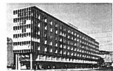
Fig. 17: KaDeWe-Passage, 1955-56 by Hans Soll. The curtain wall is made of aluminium profiles specially designed for the use of curtain wall constructions.
