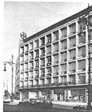
Fig. 8: Bayer-Haus, 1951-52 by Hans Geber and Otto Risse. Typical grid façade with horizontal and vertical groins showing the skeleton construction of reinforced concrete.
