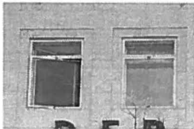
Fig. 19: Haus d. Wirtschaft, 1952-53 by Kurt Enderlein (see Fig. 6). The original steel windows could be saved by adding an extra window on the inside.
