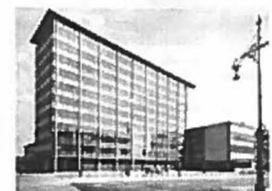
Fig. 16: Institute of Mining and Metallurgical Engineering of the Technical University, 1955-59 by Wily Kreuer. The curtain wall is based on the standardized steel window construction.
