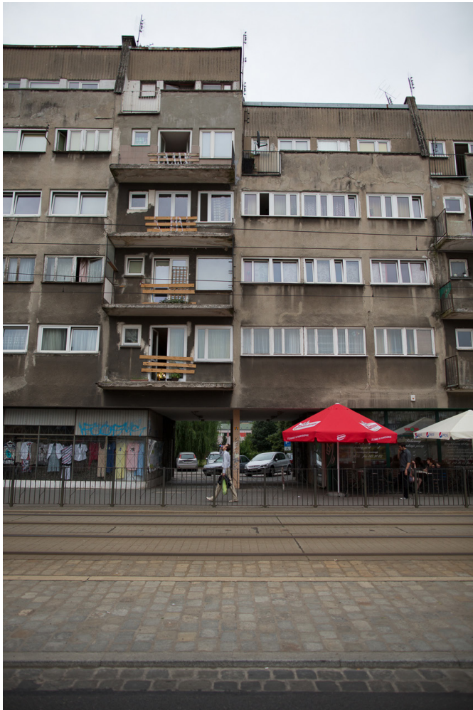
Image 6. Hazardous balconies' slabs secured by tenants
