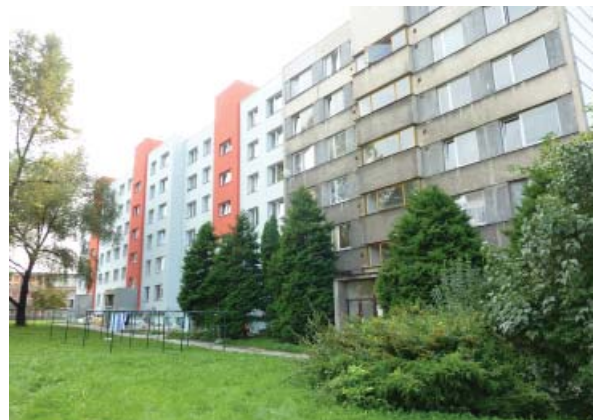
1970s panelák in the midst of renovation, Karviná-Hranice, Czech Republic. Author’s photo, 2011.
