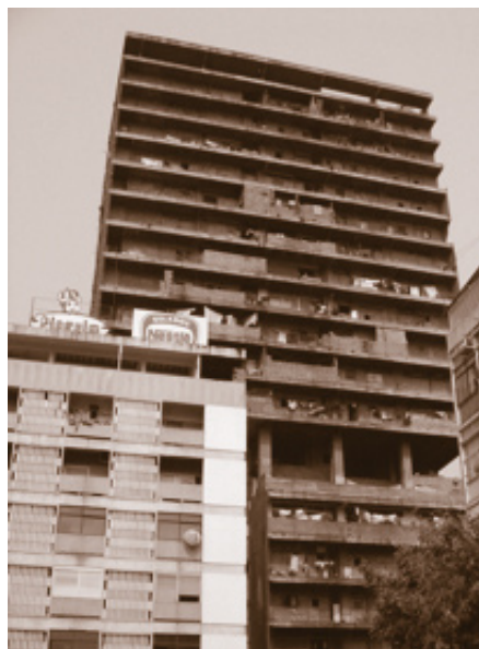
Modern high rise block in Luanda in central Luanda unfinished since prior to Independence and squatted in for decades with no services (© Paul Jenkins)
