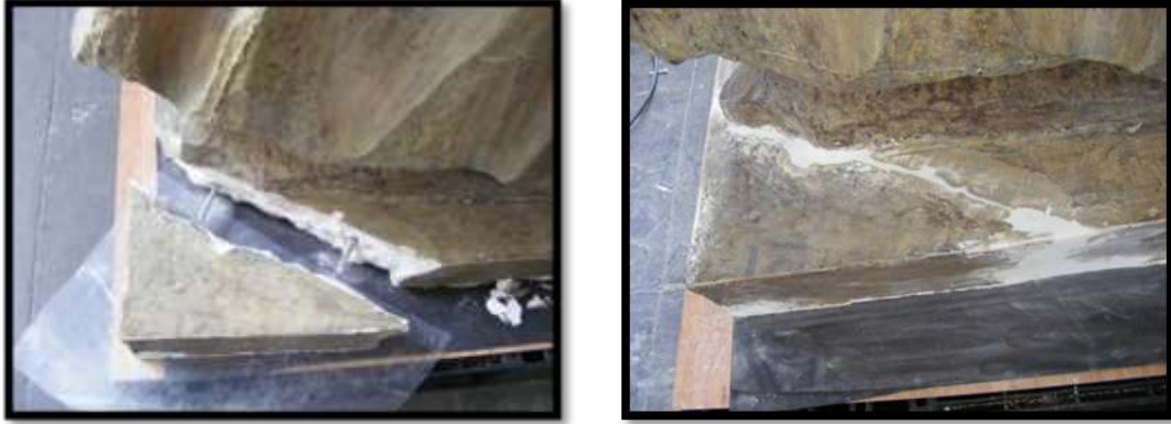
Corner of the base during repairs
