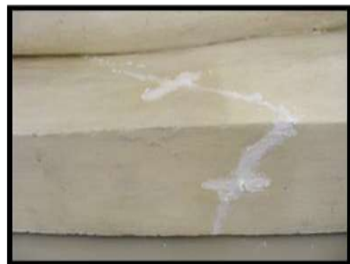
Details of the base during repairs
