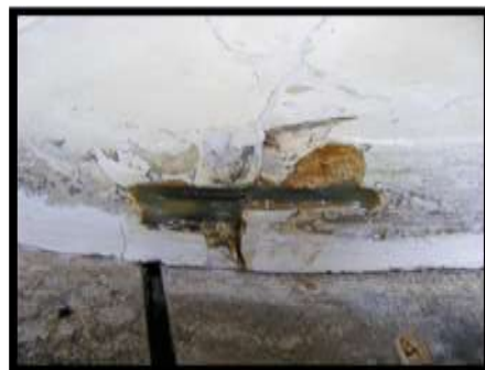
Details of fill and dowel repairs
