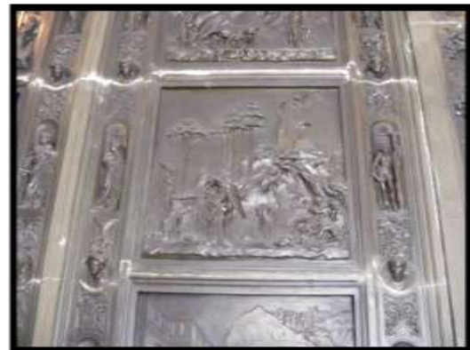
Details of fill repairs
