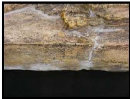
Details of fill repairs
