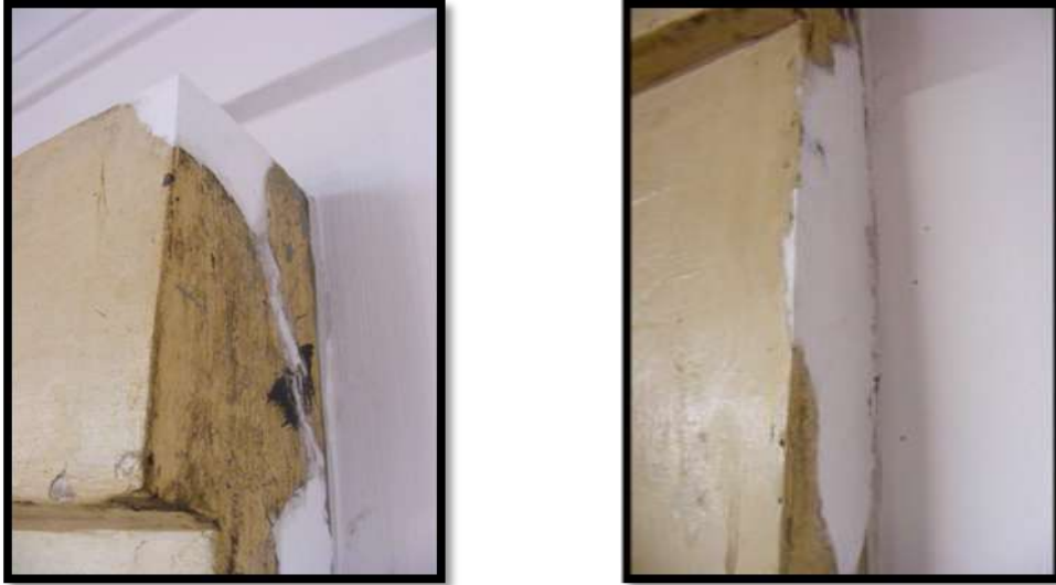
Details of fill repair
