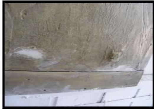
Details of fill repair
