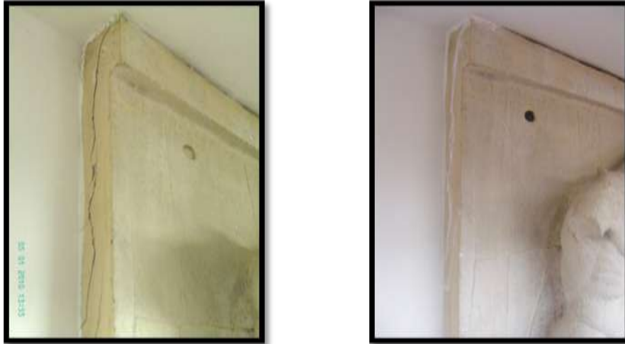
Details of fills repairs
