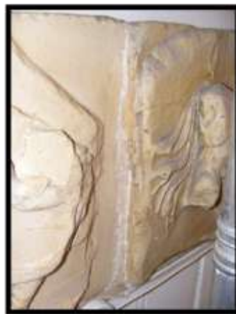
Details of fill repair
