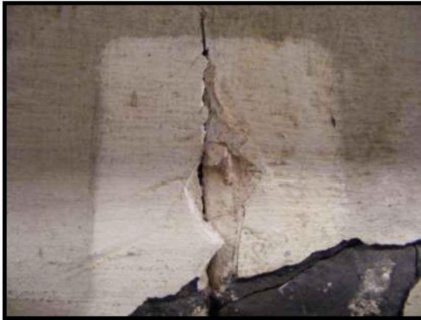
Samples of mortar were taken for analysis
