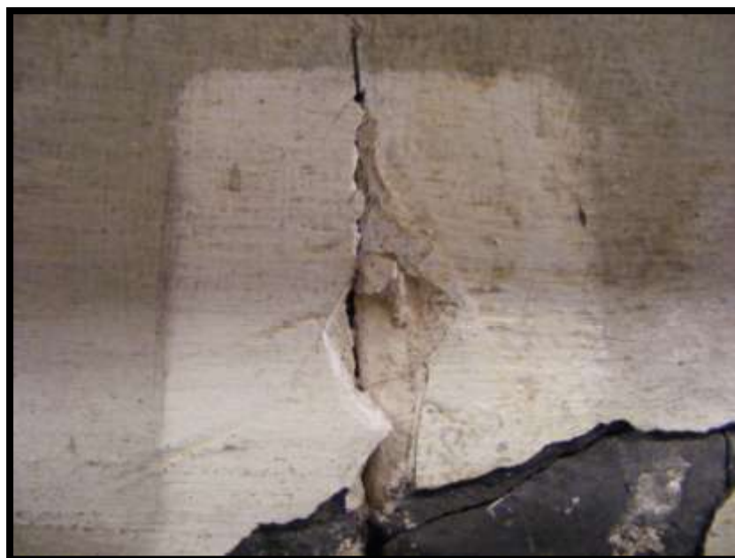
Samples of mortar were taken for analysis
