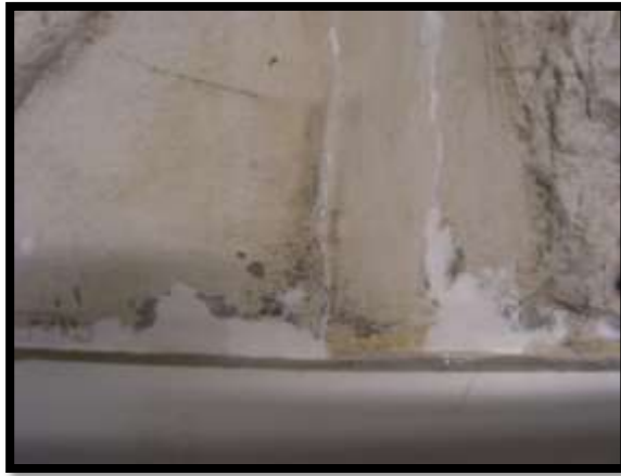
Details of fill repairs
