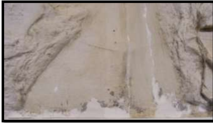
Details of fill repair
