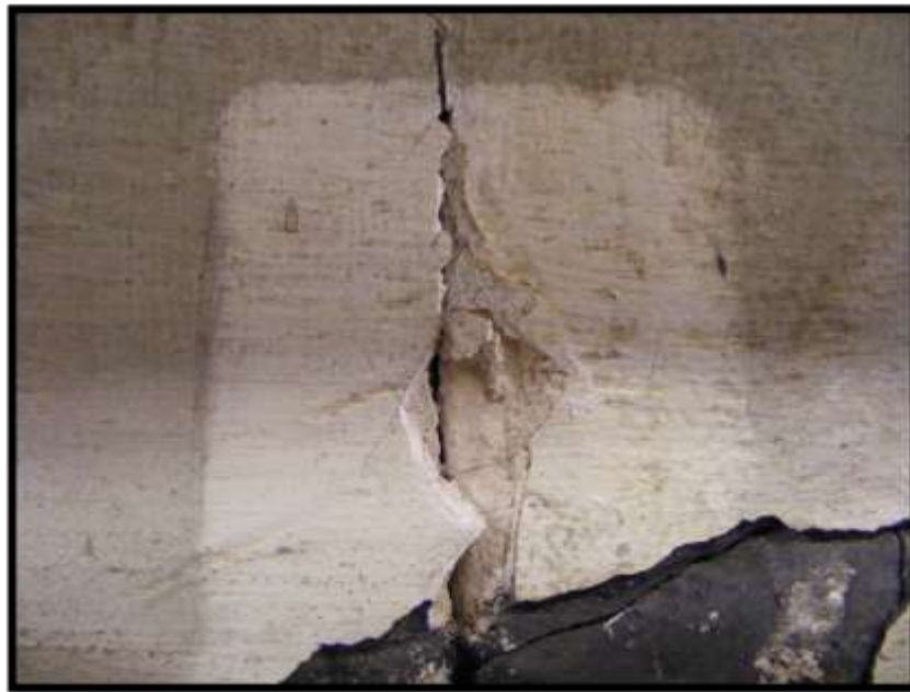
Samples of mortar were taken for analysis
