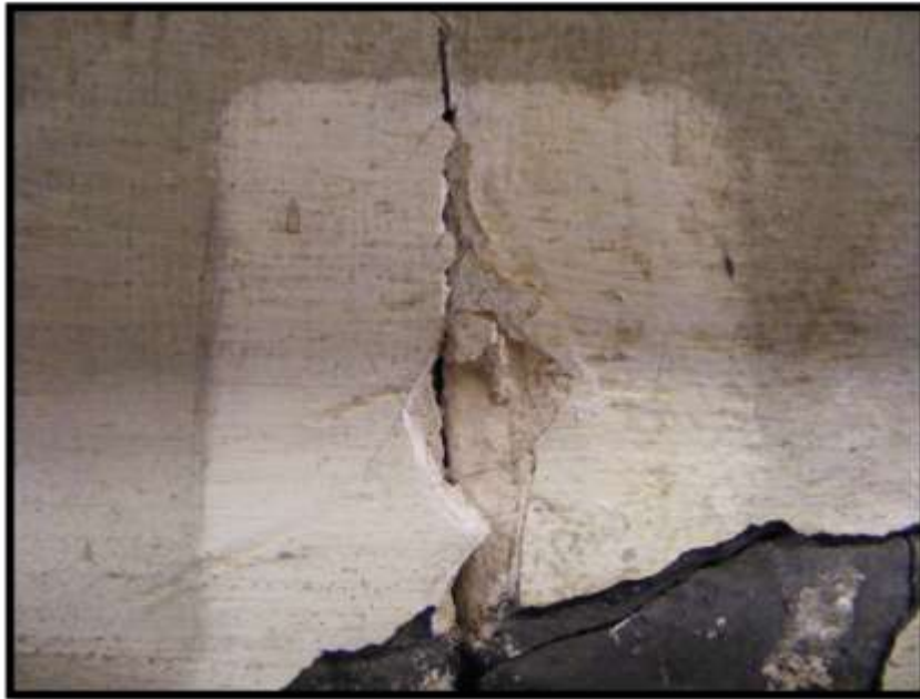
Samples of mortar were taken for analysis
