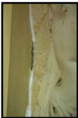
Details of fill repairs
