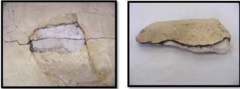
Details of repair
