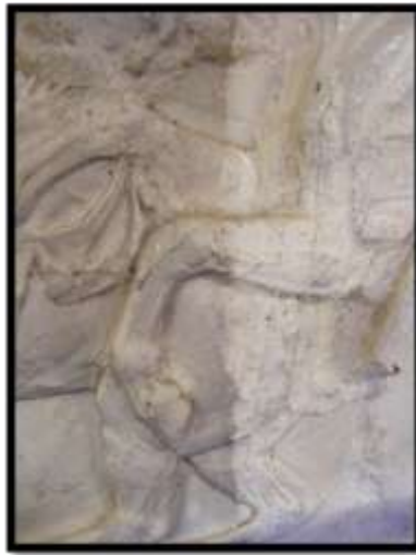
Panel during wet cleaning
