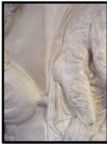
Panel during wet cleaning
