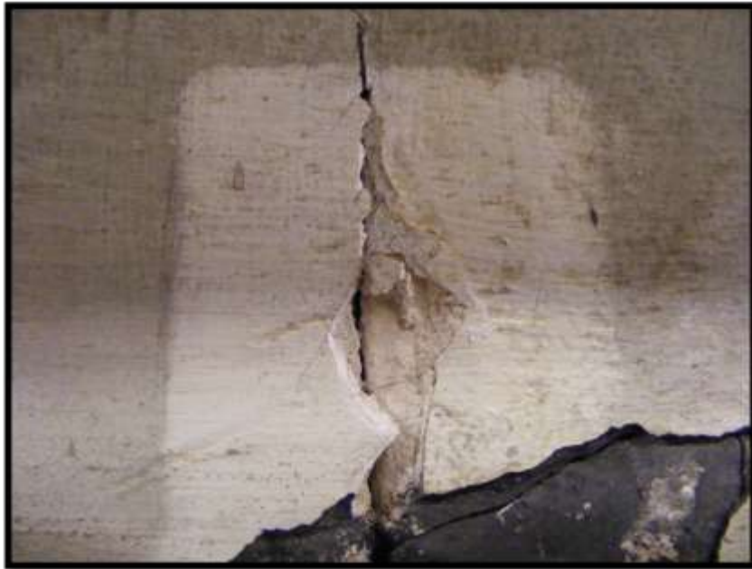
Samples of mortar were taken for analysis
