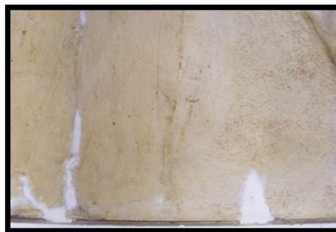
Details of fill repairs
