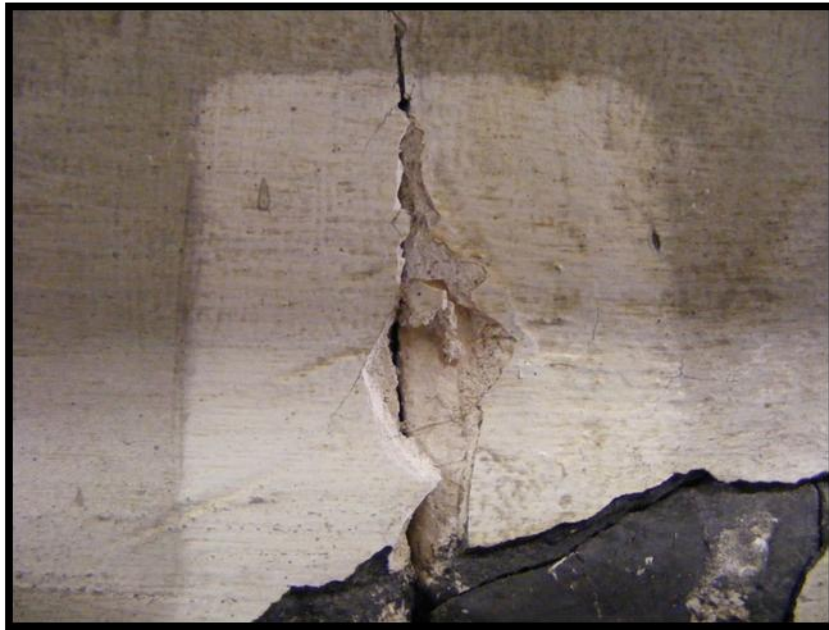
Samples of mortar were taken for analysis
