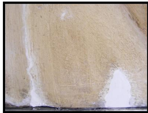
Details of fill repairs
