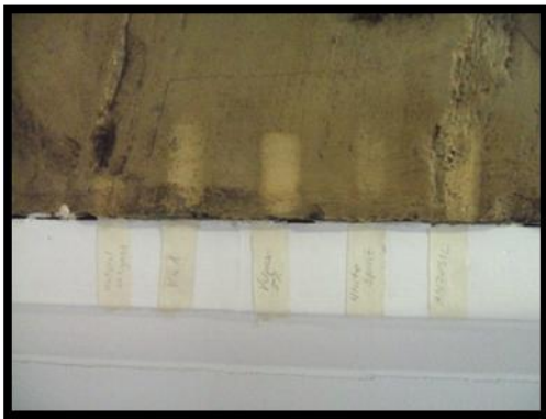
Wet Cleaning Spot Tests
