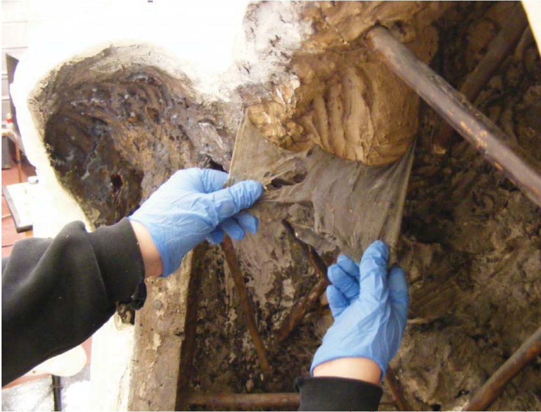
Peeling off the latex solution from the raw plaster surface
