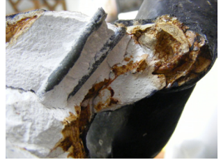
A broken foot reveals that the internal structure of the top pair of putti includes animal bone, as a very light, strong and durable material. This is not easily detectable on the X-rays due to its density being close to the density of the surrounding plaster.
